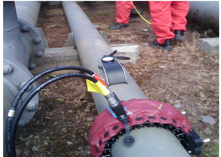
The view of the test pipe in the backward direction.
