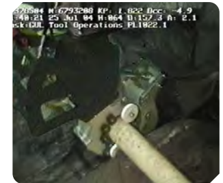
First sub-sea inspection
